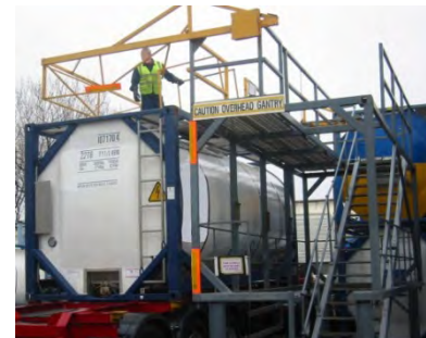
Figure 8.11 Access gantry
