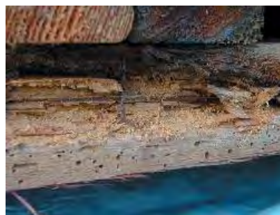
Figure 6.13 Wood frass from boring insect
