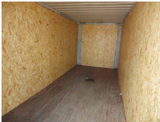
Figure 7.53 Lining a 40-foot container with chipboard panels
