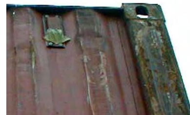
Figure 5.20 Vent tapped over
